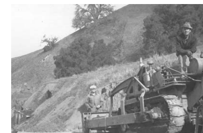
CCC crew building a road on Mt. Diablo in 1935.
